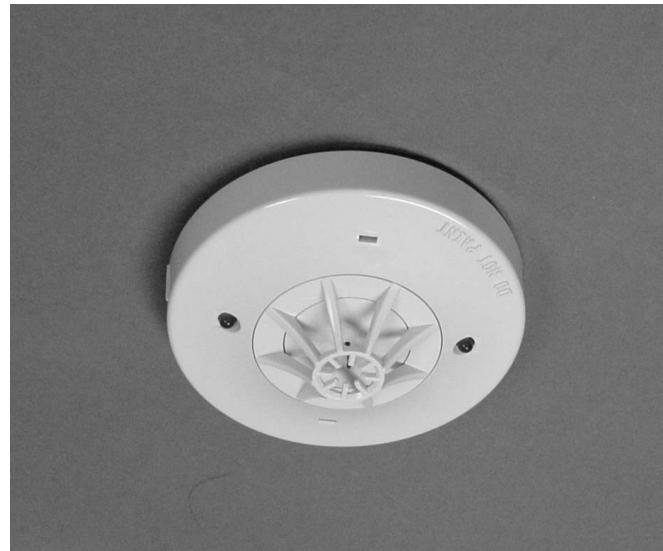
stability and transient suppression. Special signal processing techniques verify the presence of smoke before the detector will alarm.
